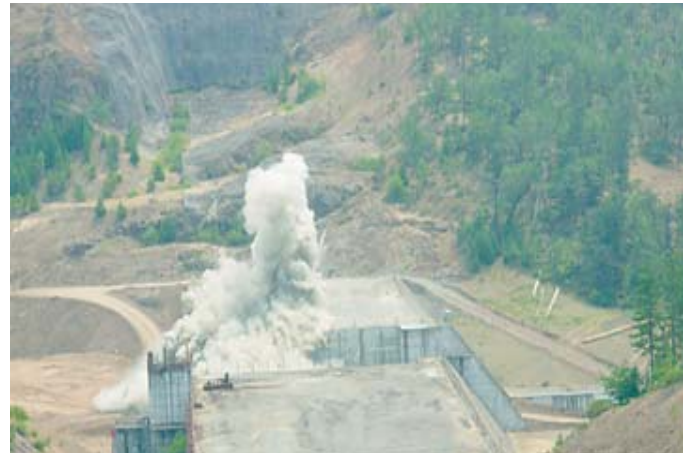
Elk Creek Dam undergoing a blast to provide salmon passage for the first time in 22 years. Photo: WaterWatch of Oregon.
